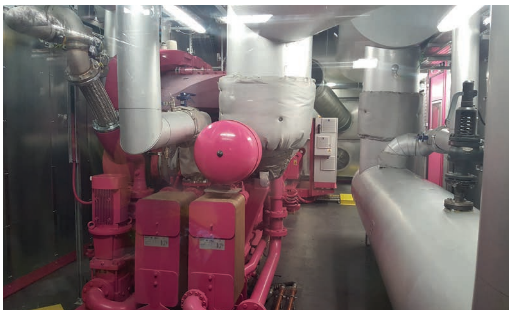
The Jenbacher pink trigen system at Barts provides a significant proportion of the hospital's heating, cooling and electricity
