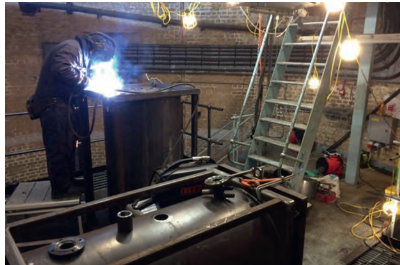
Access issues meant the boilers had to be constructed in-situ
